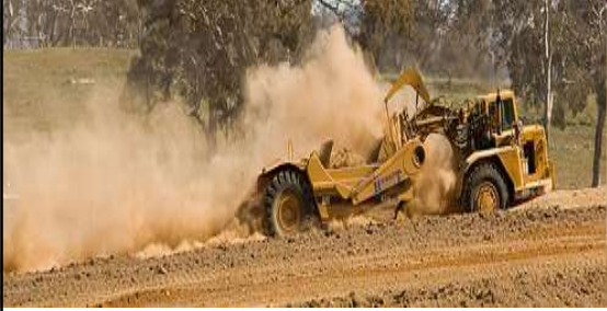
Building New Sections/Cells at the Landfill
