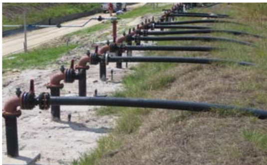
Leachate Injection Pipes
