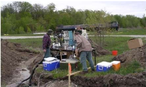
Sampling Operations at the Raw Landfill Gas Pipe Inlet
