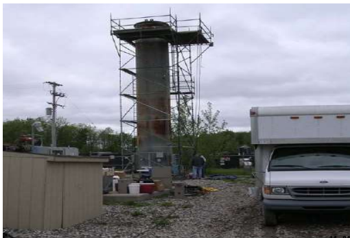
Sampling Operations at the Enclosed Flare
