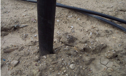
Vertical Landfill Gas Extraction Well
