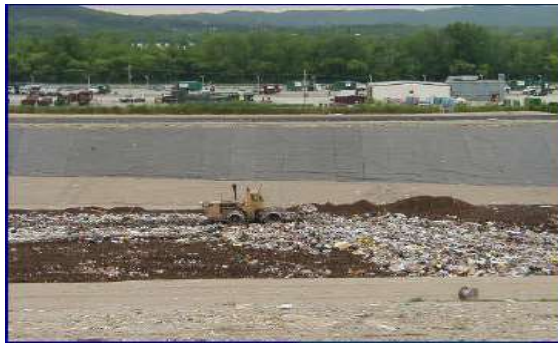
New Bioreactor Area
