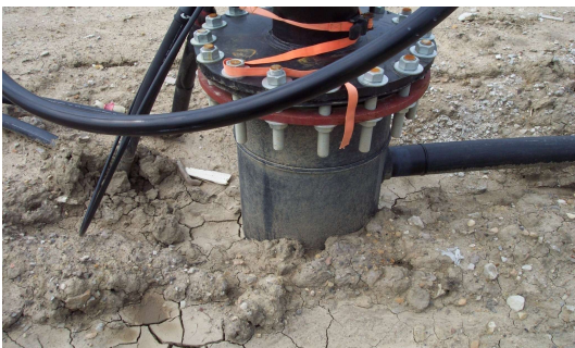
Leachate Extraction Well Riser
