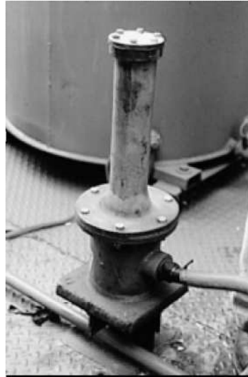
Figure 9-18. Roof-mounted rapper
