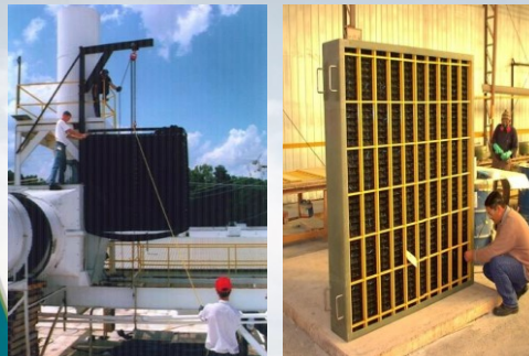
Cross-Flow Scrubber Sections
