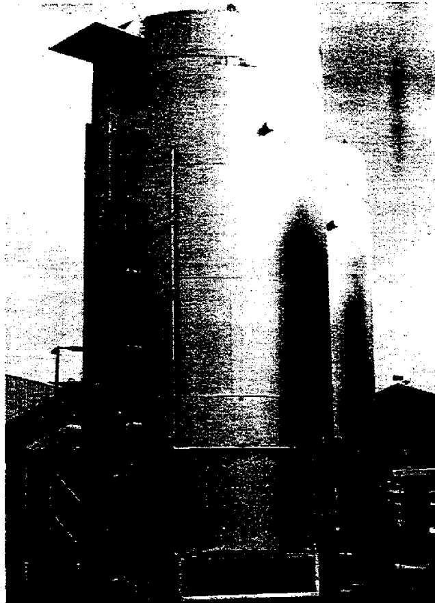
Figure 13.2 Typical Enclosed Ground Flare
