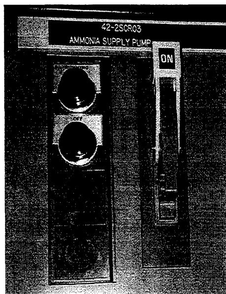
Figure 605.7 Ammonia Supply Pump Indicator Light
