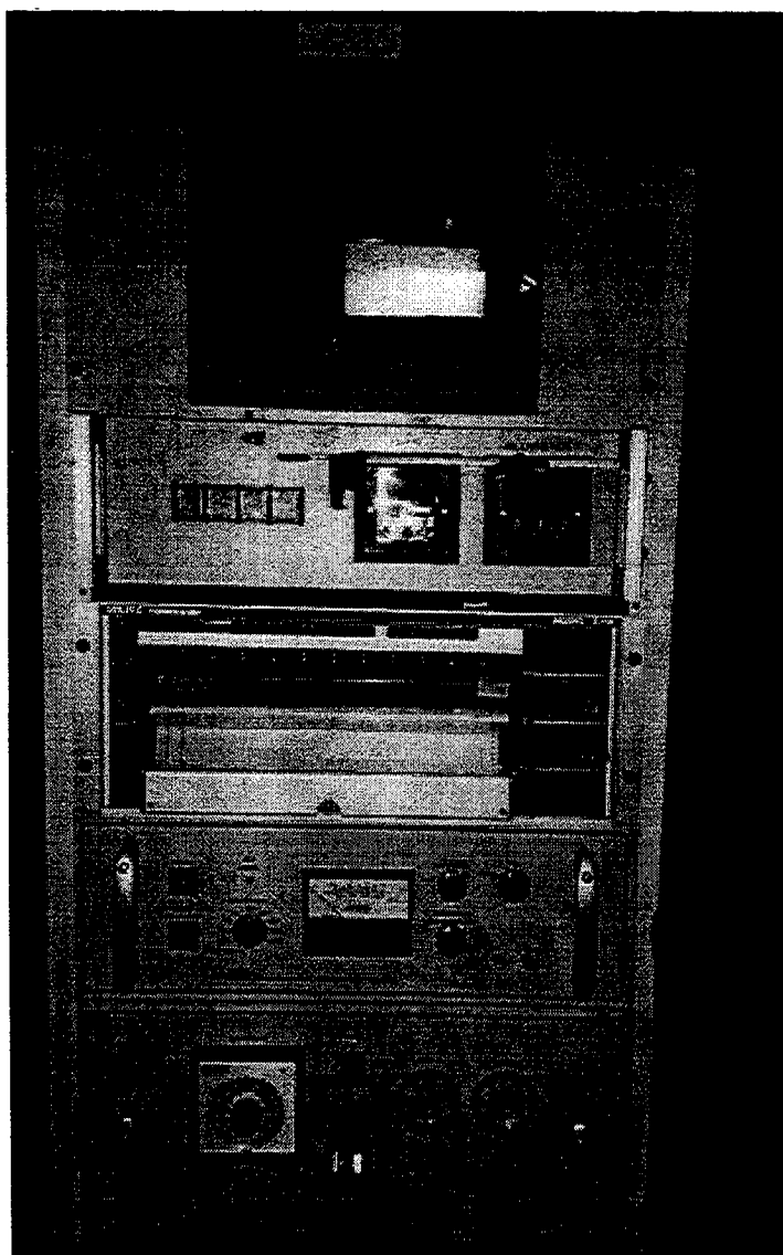
Figure 406.3 CEM Control Panel
