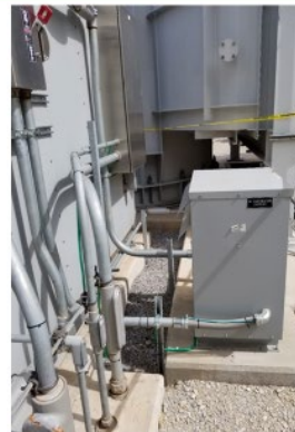
Outside a CEMS Shelter
