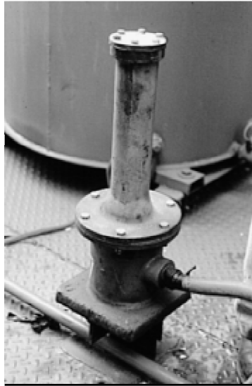
Figure 9-18. Roof-mounted rapper
