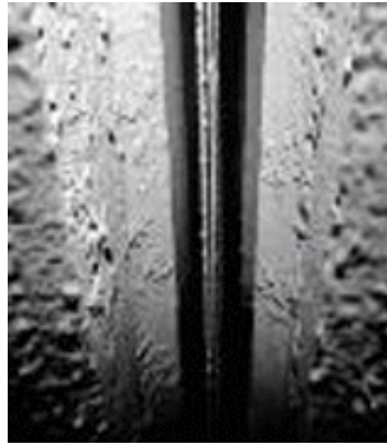
Figure 9-9. Gas passage between collection plates
