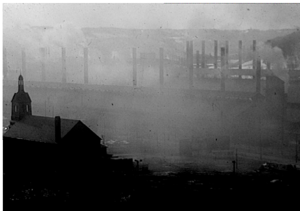
Figure 2-7. Northeast U.S. community near a steel mill, 1967
